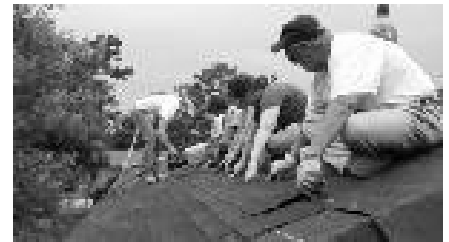
Team members lined up nailing the shingles
