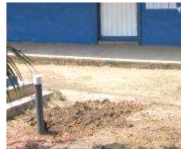
Finished well with casing installed. The next step is to add the concrete slab and put a pump on the well.
