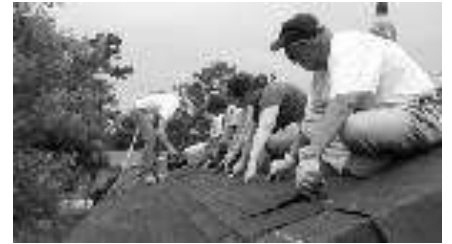
Teammembers lined up nailing the shingles
